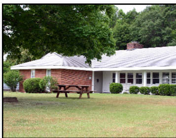
Example of residential cottage
